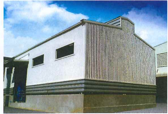
Ligman Warehouse – Chachoengsao
