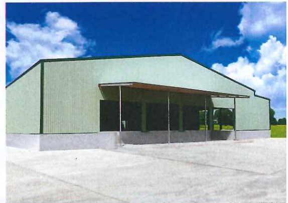
Mangoteen Warehouse - Chantaburi
