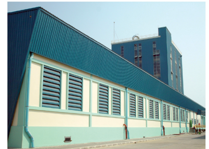
Thai Union Feed Mill 2, Samutsakorn
