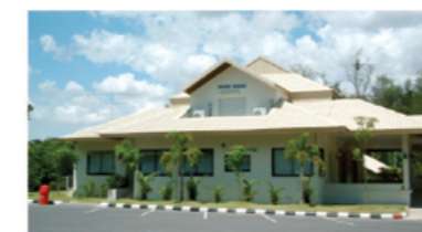
Egat Ubonrat Dam, Ubonratchathani
