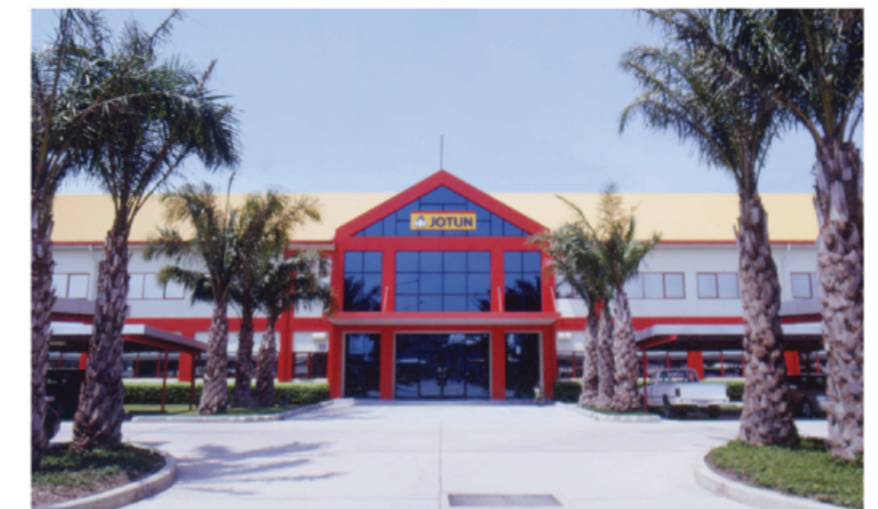
Jotun Factory, Chachengsao
