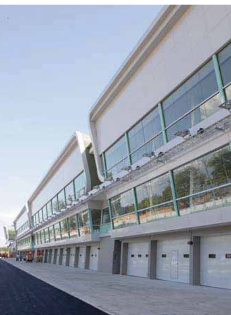
Pit Building (Photo Courtesy of Jurong International)
