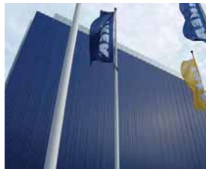
Commercial Building, Alexandra Road
