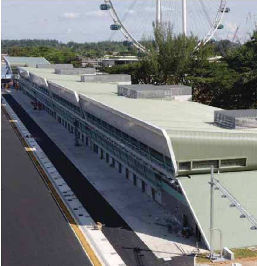
Pit Building (Photo Courtesy of Jurong International)
