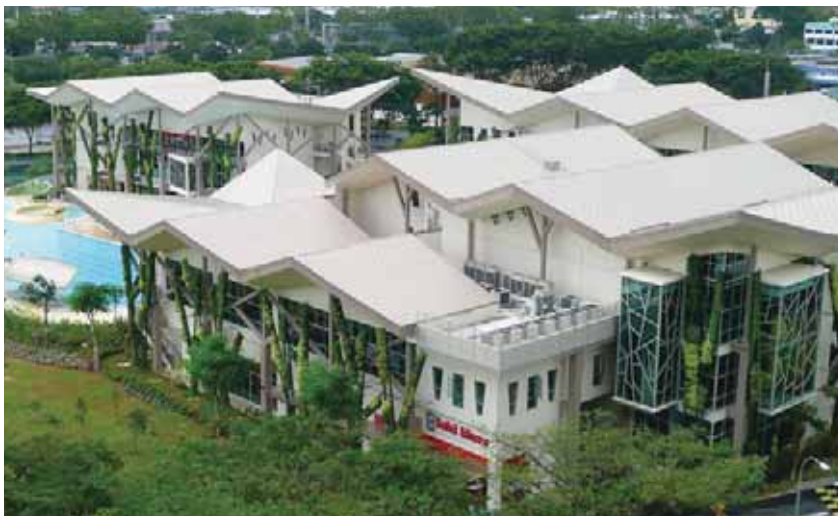
SAFRA Clubhouse @ Boon Lay
