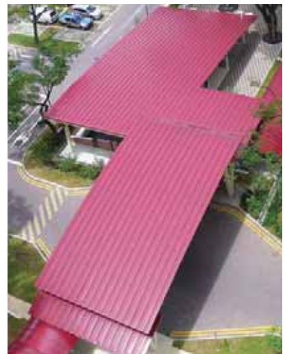
Public Housing Estate Upgrading Works
