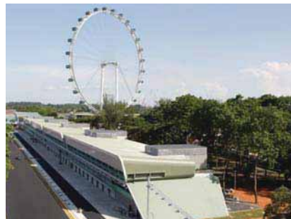
Pit Building (Photo Courtesy of Jurong International)
