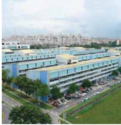
Bukit Batok Industrial Park (Re-roofing Works)
