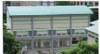
Indoor Sports Hall, School Upgrading Programme, Fuhua Secondary School
