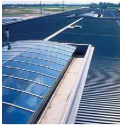
Changi International Airport, Terminal 2
