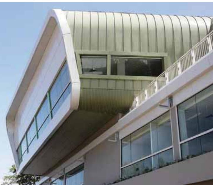
Pit Building (Photo Courtesy of Jurong International)
