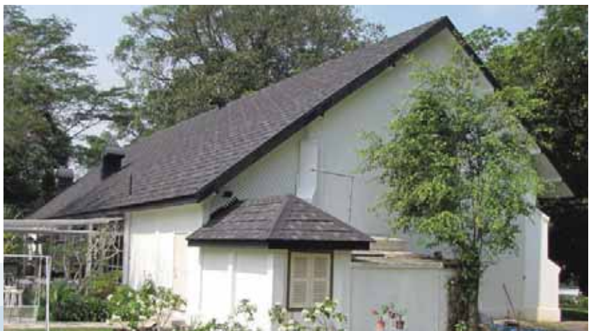
Commercial Establishment, Harding Road
