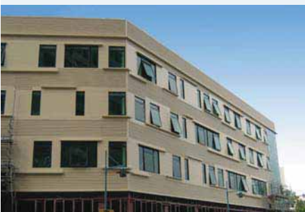
Tan Tock Seng Hospital (Extension Building)
