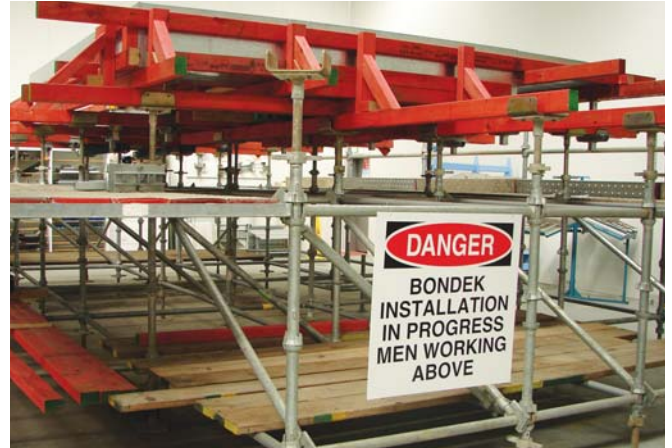
Step 2: Place props if required
