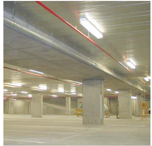
Step 11: Allow slab to cure and remove props
