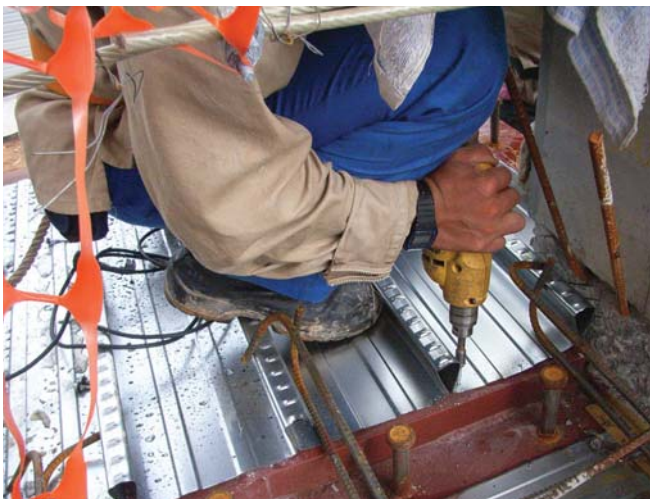
Step 5: Fix BONDEK® II sheets to steel beams
