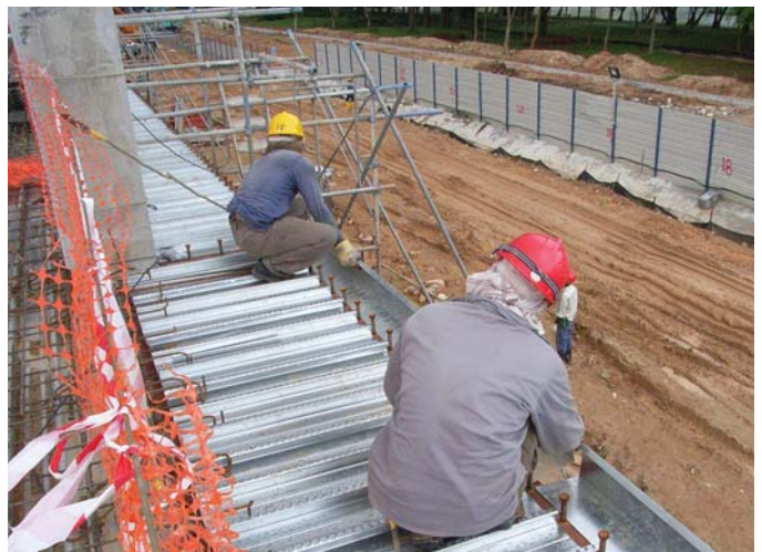
Step 6: Install Edgeform
