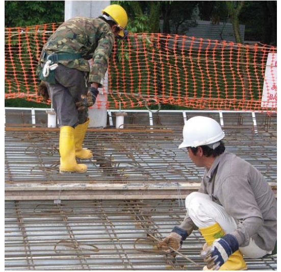
Step 8: Place steel reinforcement bars
