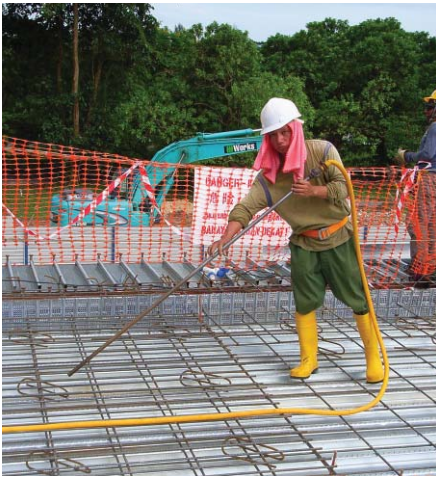
Step 9: Remove dirt and contaminants
