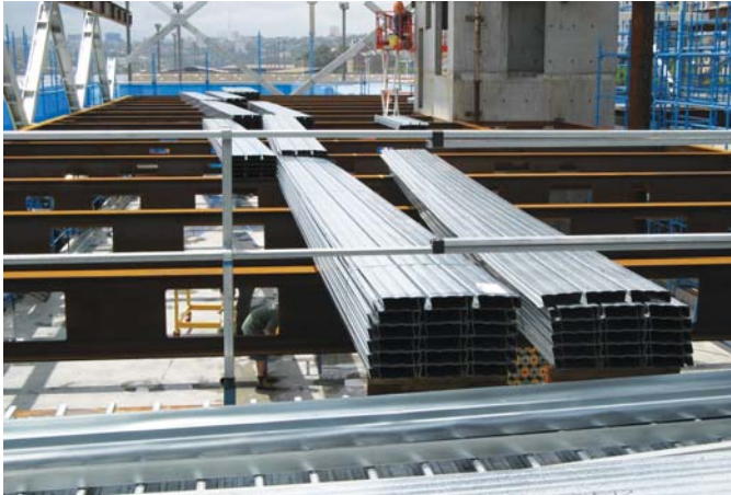
Step 1: Place BONDEK® II sheet bundles on support
