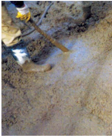
Step 10: Place concrete
