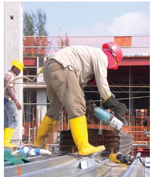
Step 4 - Trim BONDEK® II sheets, if required
