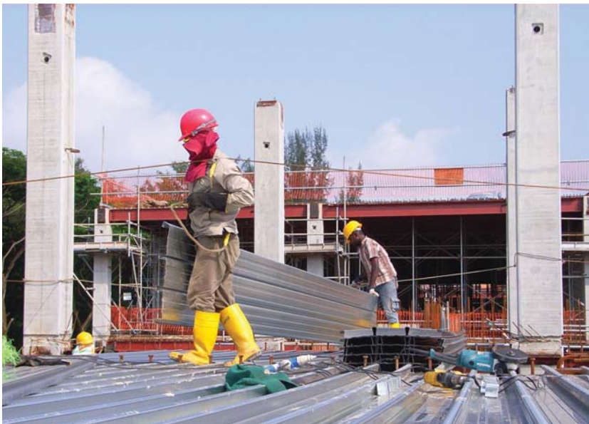
Step 3 - Lay BONDEK® II sheets
