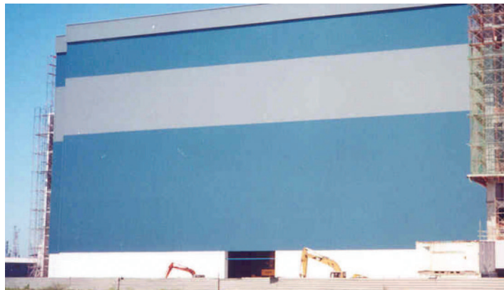
PTC Warehouse, Singapore
