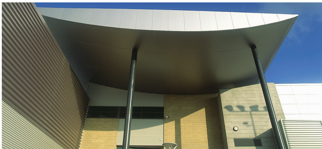
Wall Application, Project in Australia
