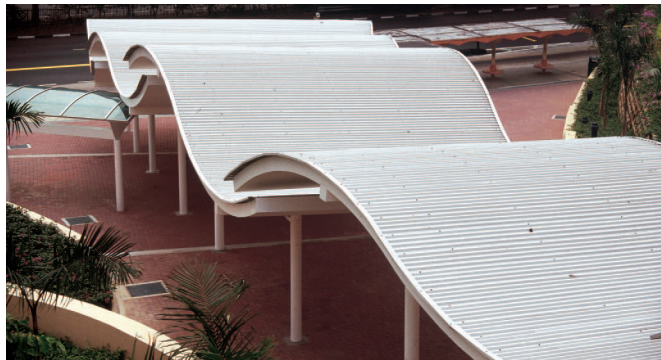
Linkway at Queensway, Singapore
