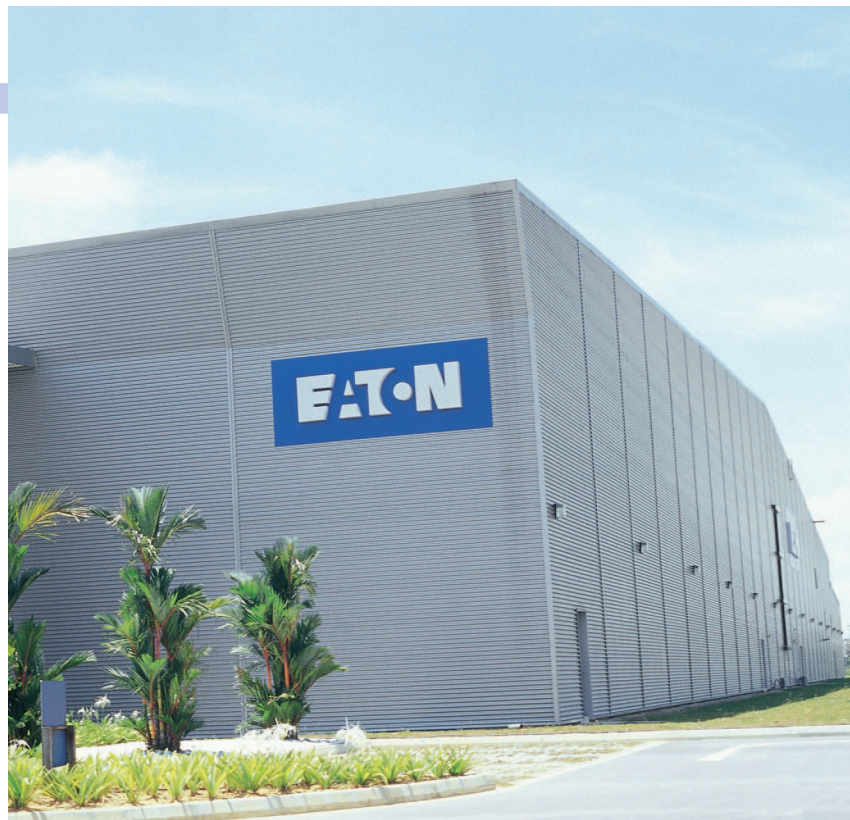
Eaton Building, Singapore
