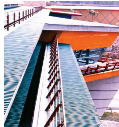
Project in Malaysia
