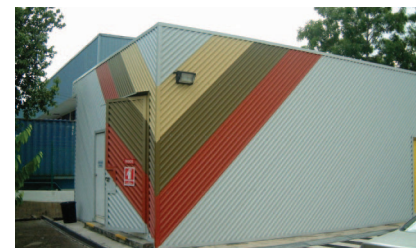
Sub-station at BlueScope Lysaght, Singapore
