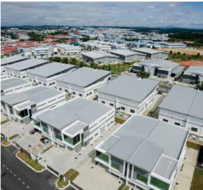
Frontier Industrial Park, Johor
