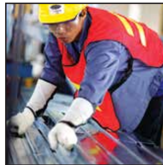
Can be fabricated off-site and delivered pre-assembled
