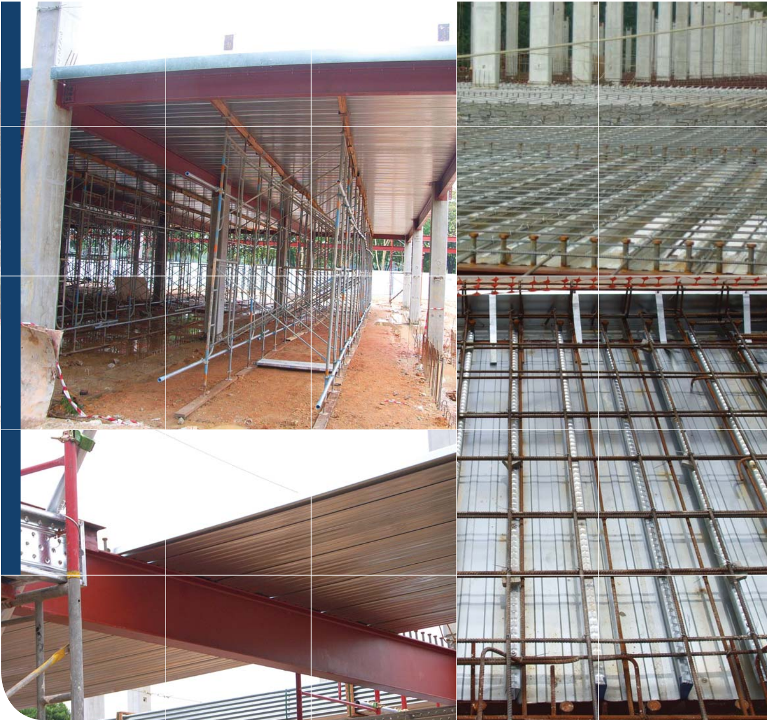
Fig 6.2 Installation of LYSAGHT® structural steel decking systems
