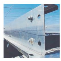
Lysaght® Zed and Cee sections are accurately roll-formed from high-strength zinc-coated steel to provide an efficient, lightweight, economical roofing and cladding support system for framed structures.
